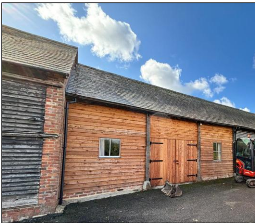
Clad building adjacent to open bays
