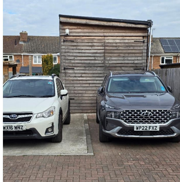
Outbuilding workshop from the access lane
