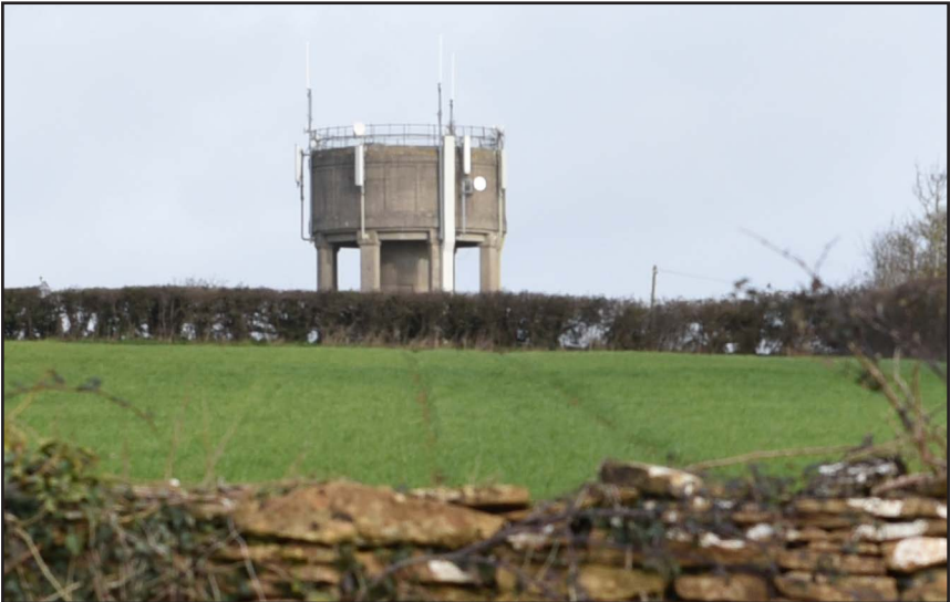
The water tower occupies a high point near the Site and Sherston and, as a result, forms a prominent reference point within the Study Area.
