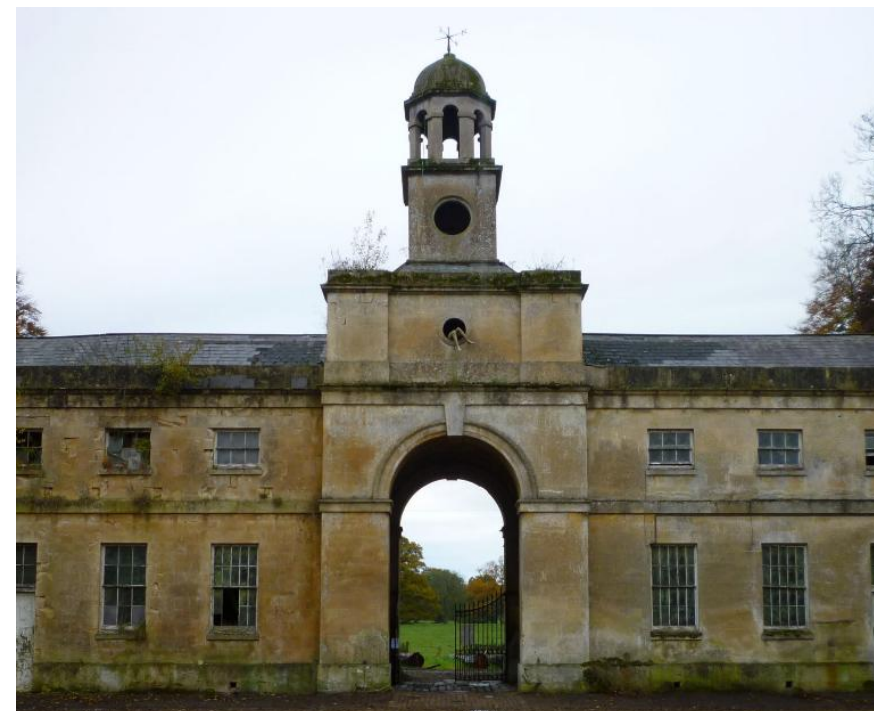
Figure 2. Stables Entrance circa 2016 (Marlborough.news).
