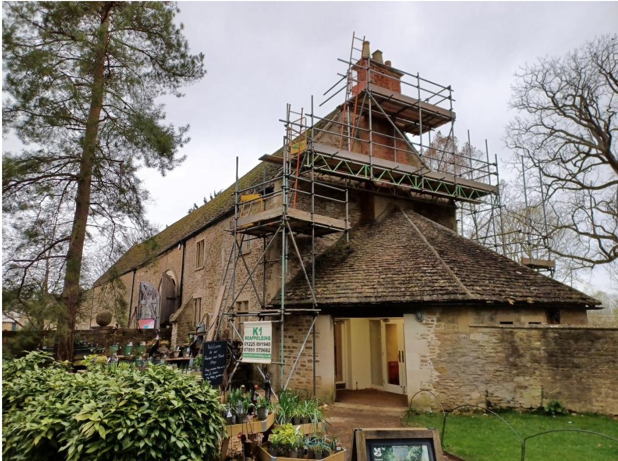
Image 1: Overview of Gable elevation showing location of chimney and single story extension with main visitor rout into Lacock Abbey Grounds beneath the stack.
