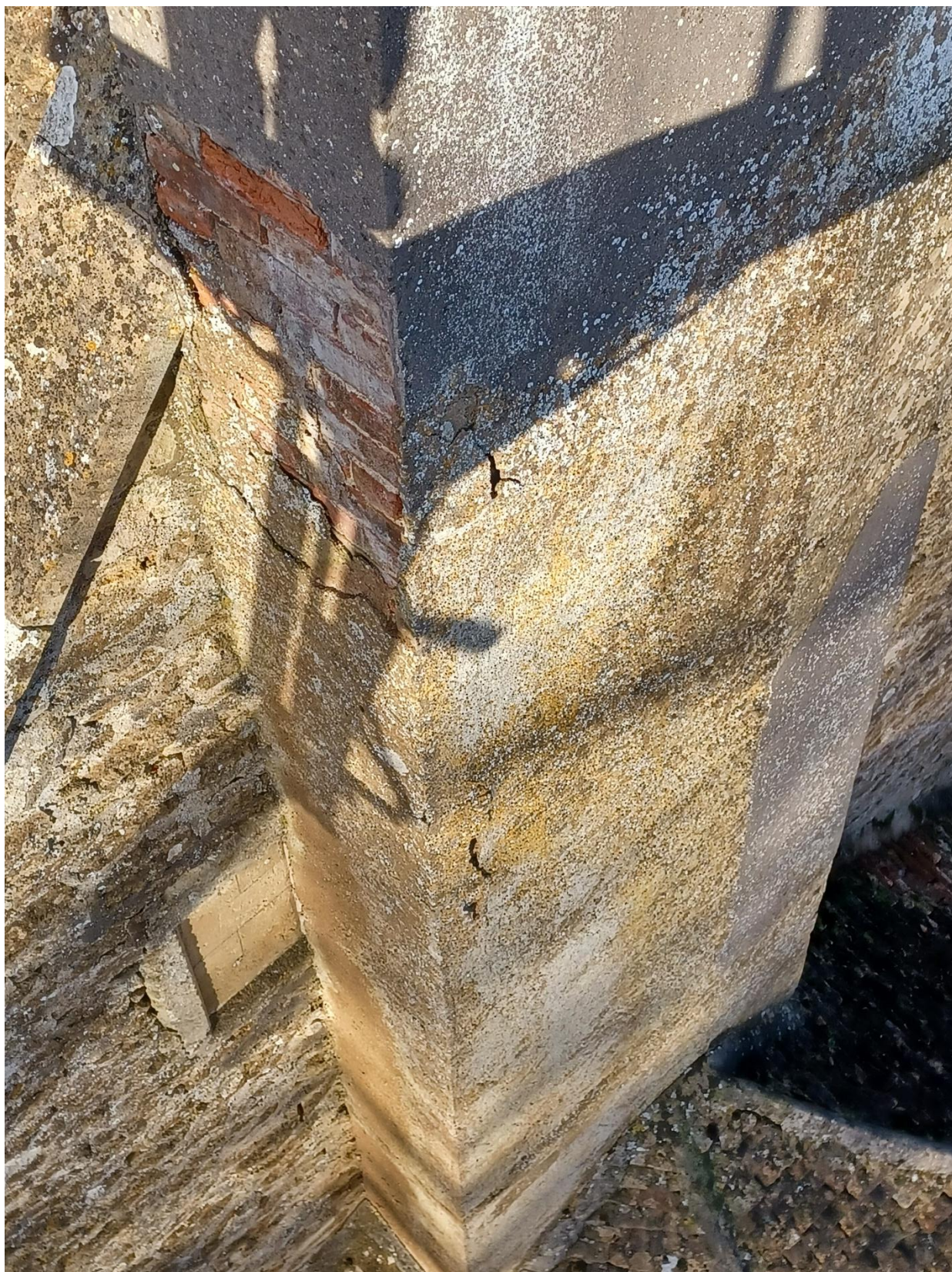
Image 5: showing loss of render and differing renders across stack.
