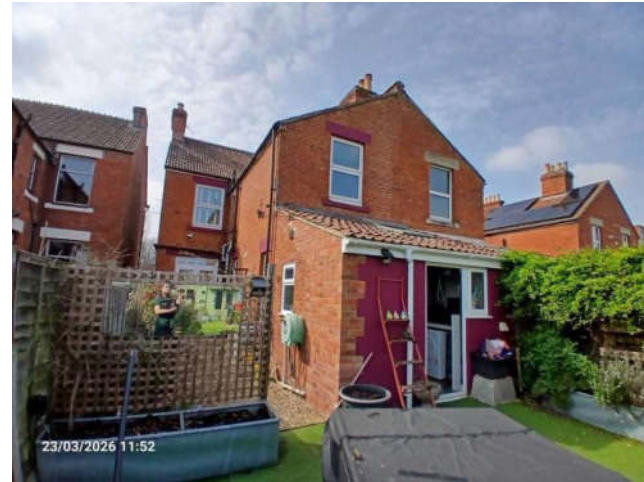
Photo 10: Southeastern and northeastern elevations of B1.
