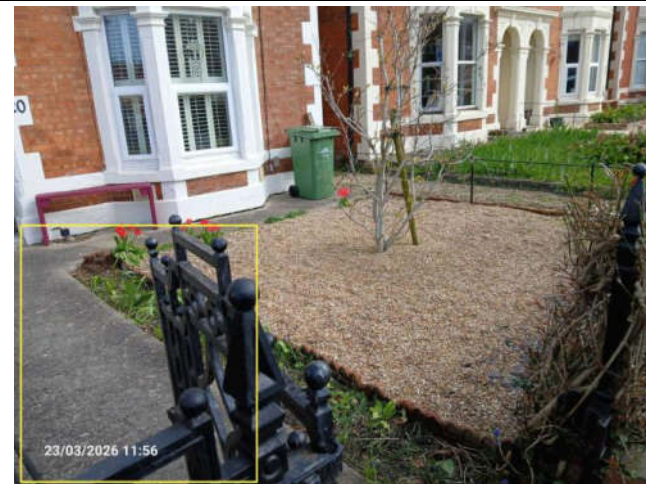
Photo 4: Small concrete access path in front of B1.
