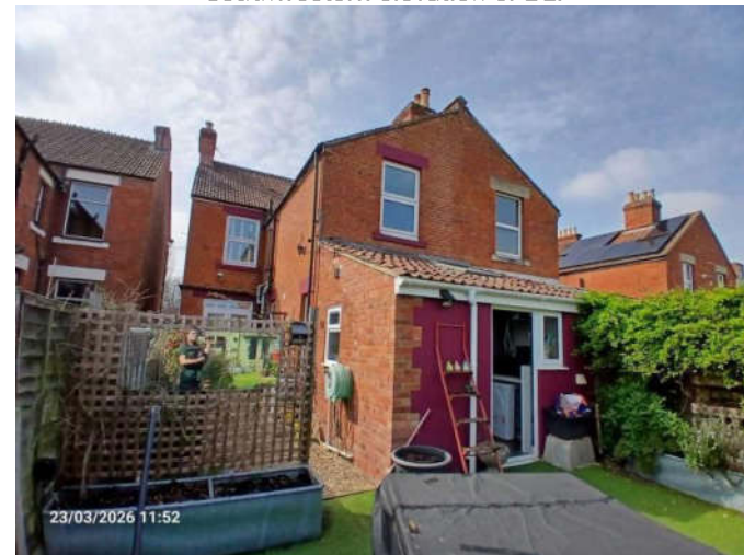
Southeastern and northeastern elevations of B1.
