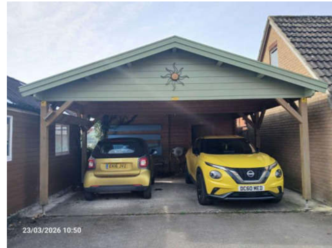
Northeastern elevation of B4 and the adjoining carport.
