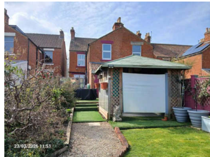
Southeastern and northeastern elevations of B2.
