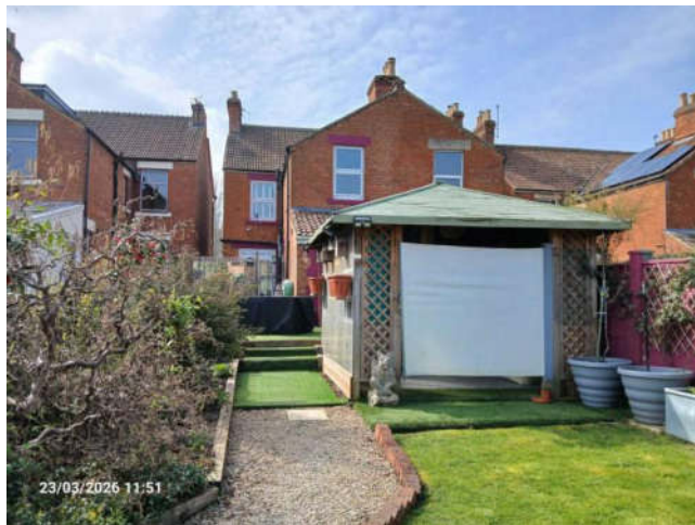
Photo 11: Southeastern and northeastern elevations of B2.
