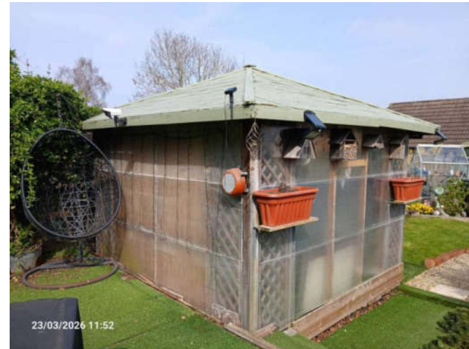
Southeastern and southwestern elevations of B2.
