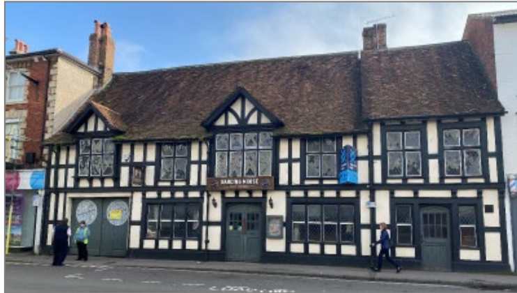
Figure 2 - Front facade facing Castle Street
