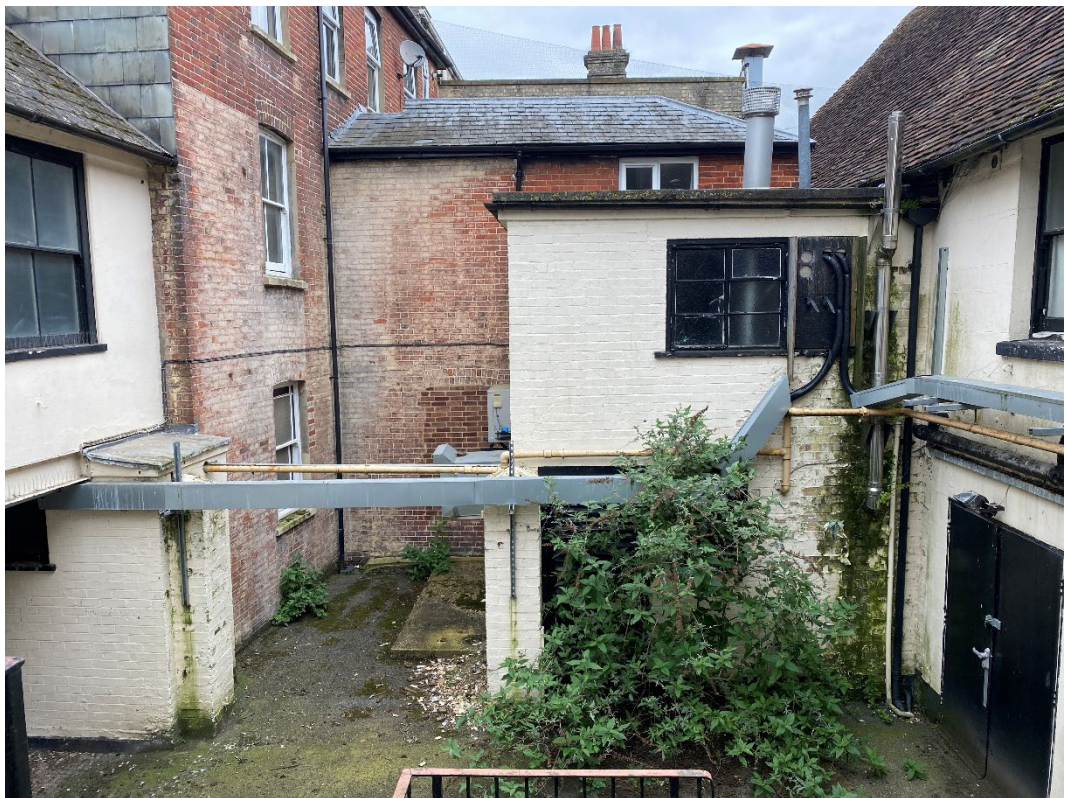
Figure 11: The northern yard, arch to Castle Street on left, former stable range on right.
