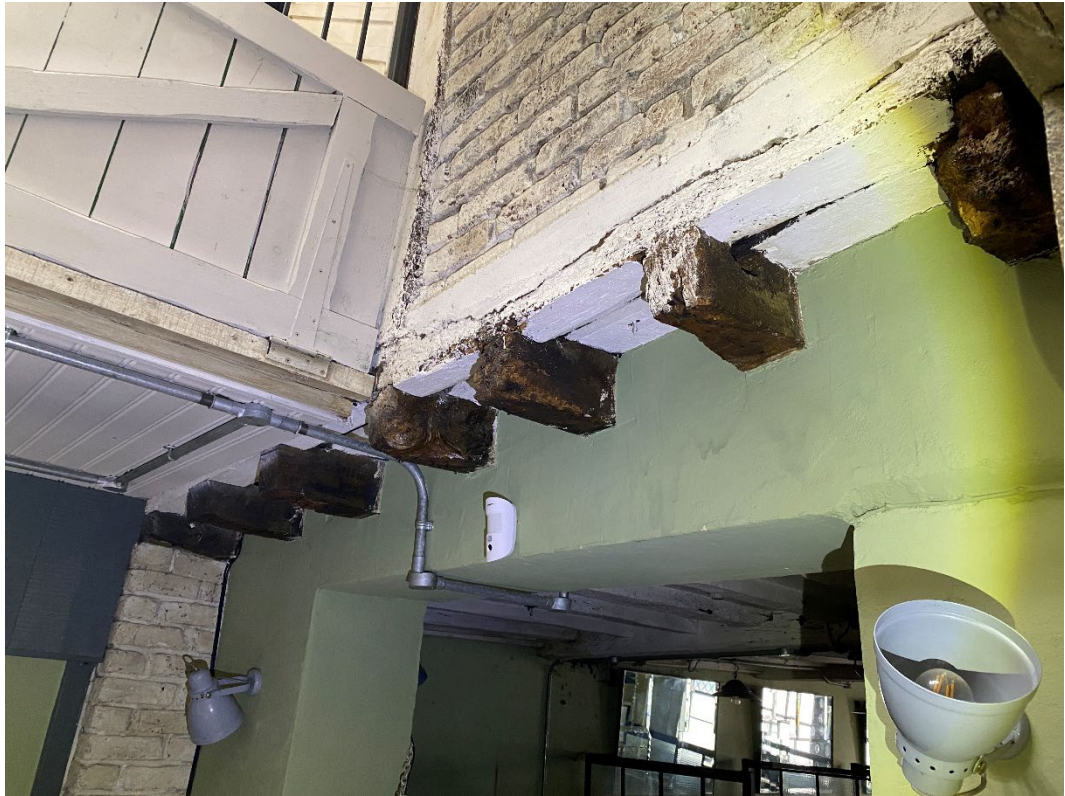
Figure 16: Retained external jetty of the south western structure, probably 16 th century, now enclosed within the central linking structure.
