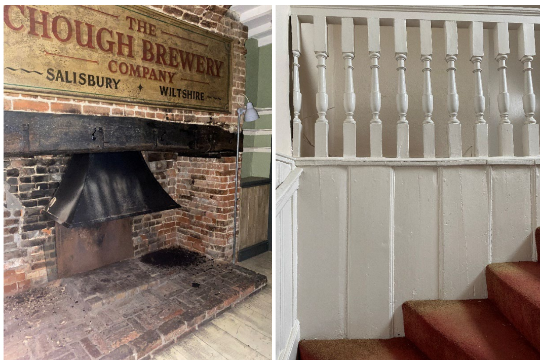
Figure 18-19: (Left) large open fireplace in the rear part of the eastern range; (right) stair balustrade and historic panellled wall at attic level.
