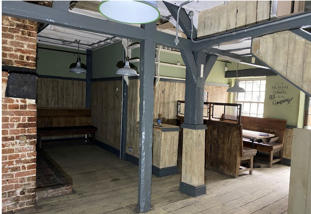
Figure 23: The southern end of the western range, large stack on the left and in the centre the intruding fire escape compartment hard against the historic window. Removal will reinstate this floor plan.
