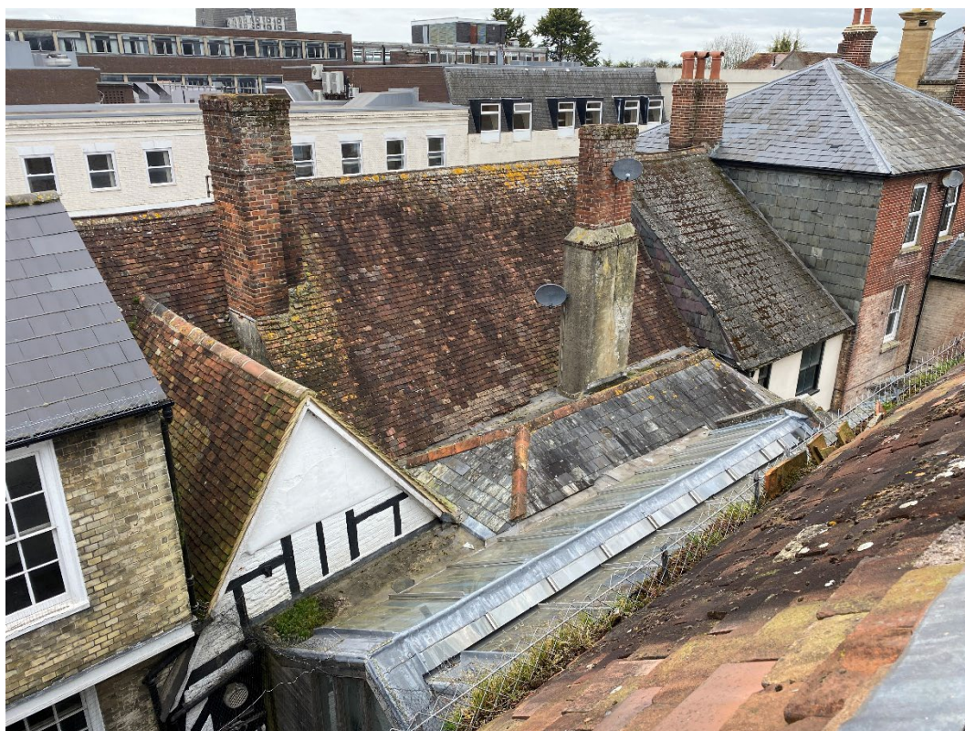
Figure 13: the roof scape of the central and Castle Street ranges. Note timber framed gable to left.
