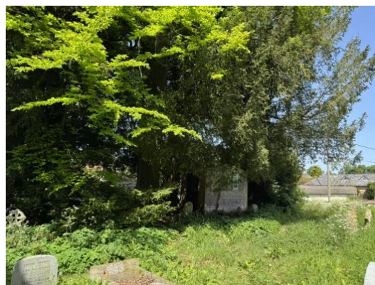
View from the churchyard to north of church. Existing/proposed shed beneath the trees.
