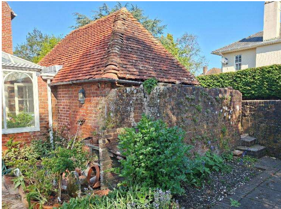
Figure 13 The screening wall to the east of the outbuilding.
