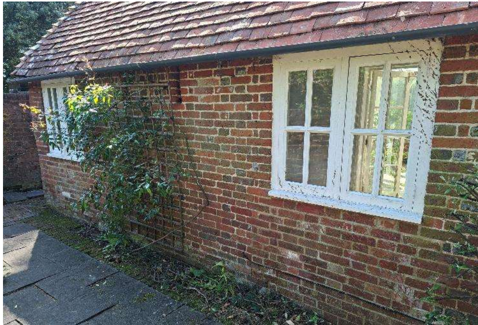
Figure 10 North elevation of the outbuilding with two modern windows infilling former doorways.
