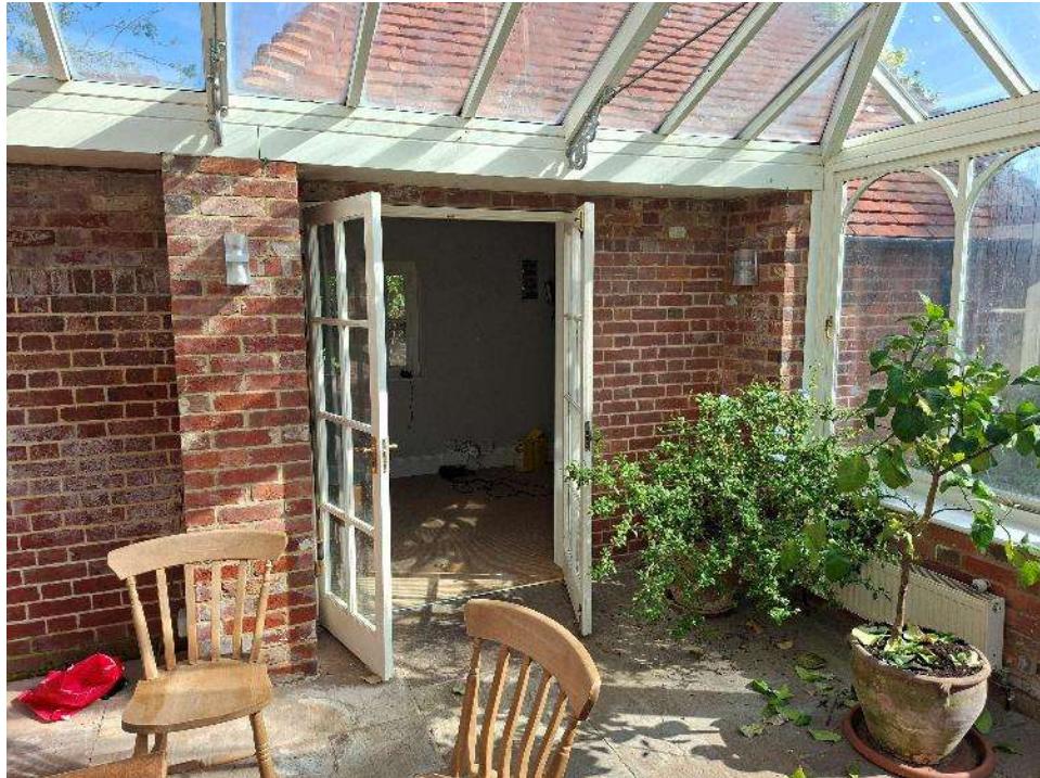
Figure 14 The modern entrance to the outbuilding from the conservatory, with rebuilt brickwork to the right.
