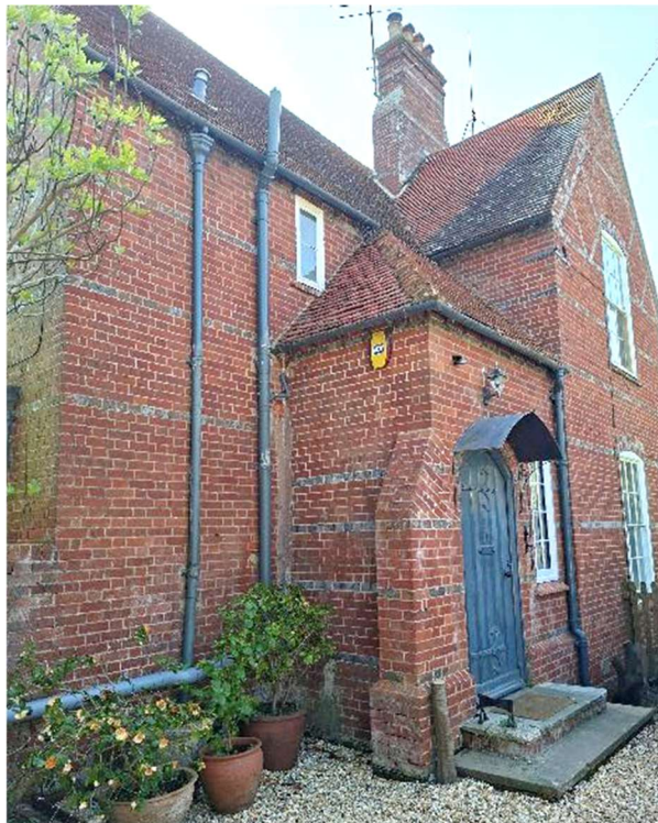
Figure 6 Front, west elevation.
