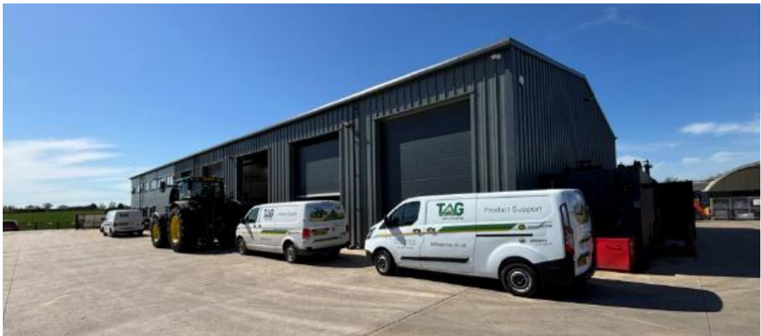
Figure 2: Existing dealership/workshop building
