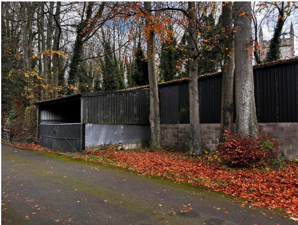
Figure 2 - Photograph of the barn
