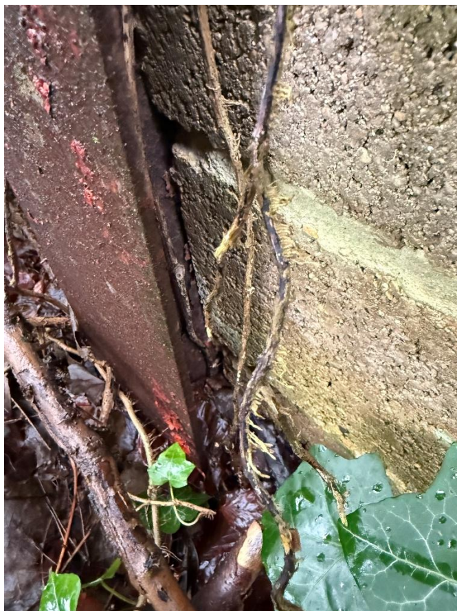
Figure 12: Steel Corrosion 2, South-east Elevation
