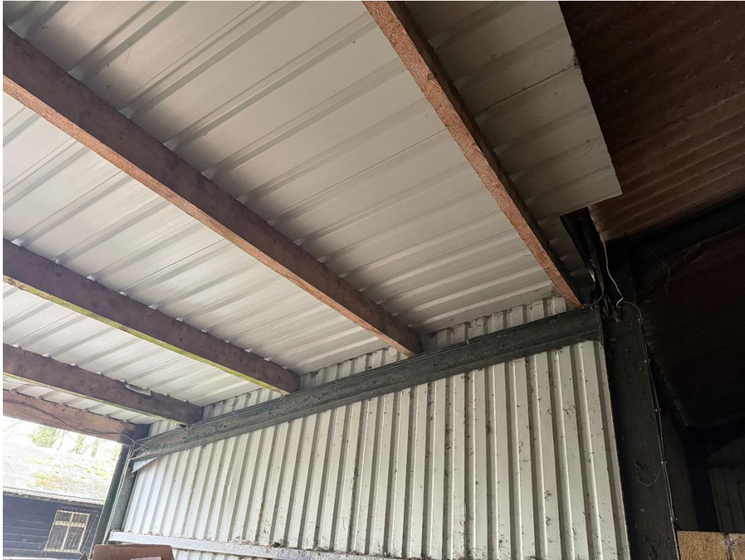
Figure 10: Steel Corrosion 1 – Top of masonry internally
