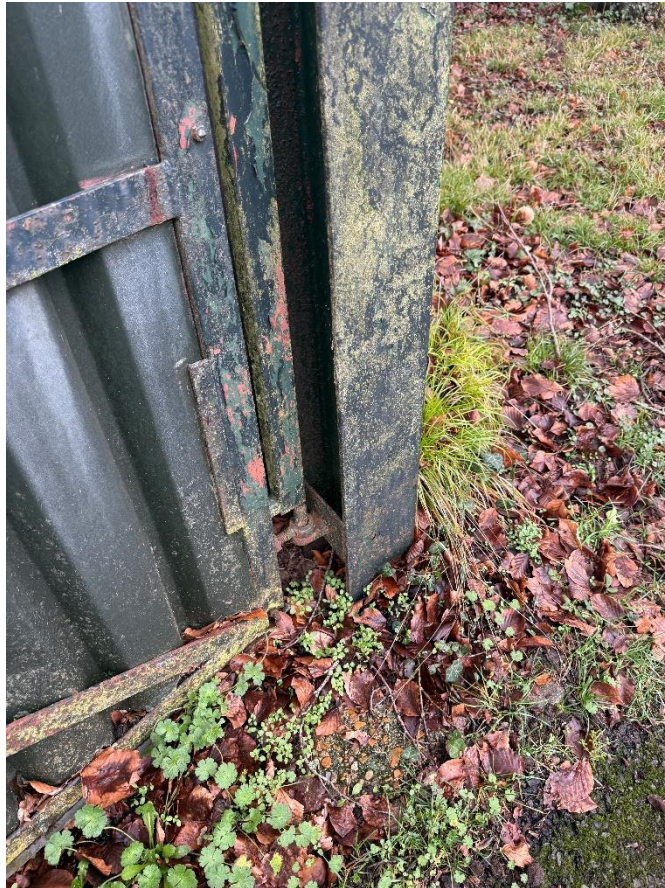
Figure 12: Steel Corrosion 2, South-east Elevation
