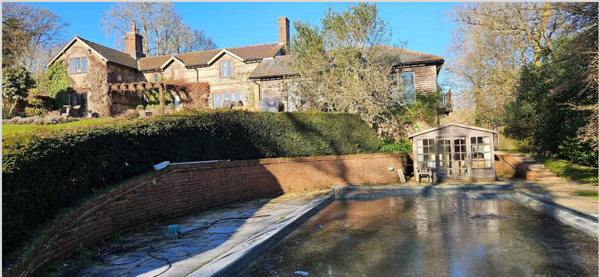
Above: Existing rear elevation, pool house and swimming pool
