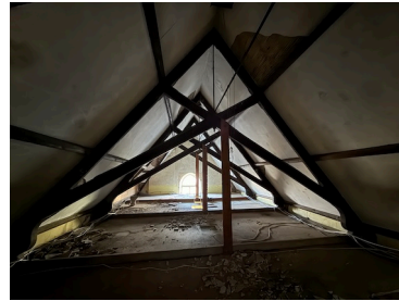
Fig 20 – Roof Void / Large Hall: Truss Configuration & Scissor Bracing
