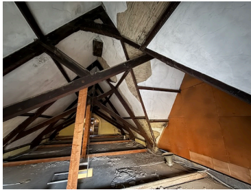
Fig 19 – Roof Void / Large Hall: King Rod Scissor Trusses (Hidden by False Ceiling)
