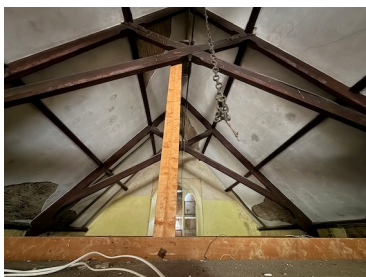
Fig 23 – Truss Detail: King Rod & Scissor Bracing Showing Wrought Iron Construction
