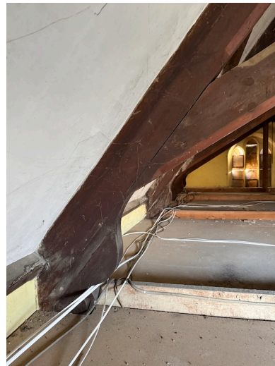
Fig 22 – Truss Detail: Rafter with Stop-Chamfered Victorian Carpentry
