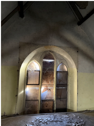
Fig 21 – Roof Void / Large Hall: Blocked Stone Mullioned Window (Proposed Restoration)
