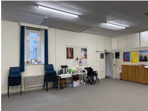
Fig 1 – Large Hall: False Ceiling Concealing Victorian Roof Structure
