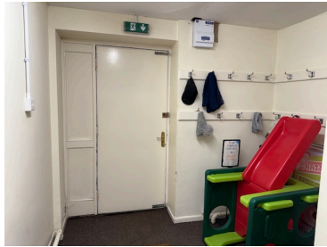
Fig 7 – Entrance Hall: Existing External Door & Lobby
