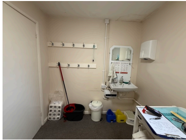
Fig 13 – Female Toilet: Existing Washbasin Area
