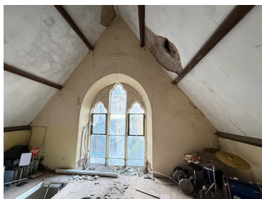
Fig 17 – Roof Void / Toilet Block: Victorian Timber Roof Structure
