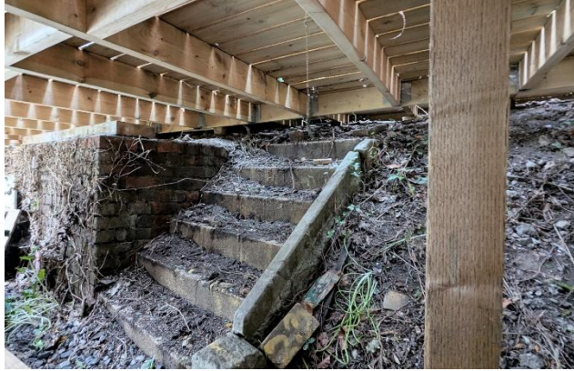
Fig. 6 View of structures and levels retained in situ under decking.
