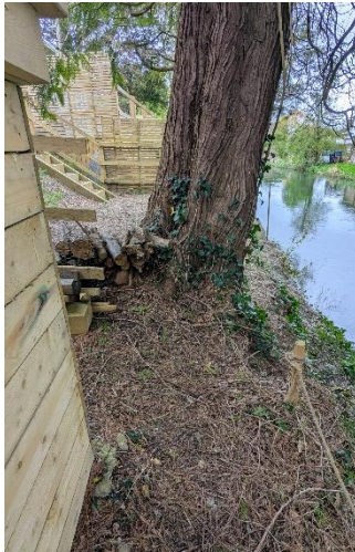
Fig. 7 View east showing T3 in relation to the decking. Note: post-hole at the corner of the structure (visible bottom-left in this picture) was lined with impermeable lining before backfilling with concrete
