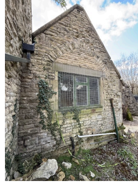
Fig 8 – NE Elevation: Kitchen at River Marden Boundary
