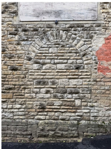
Fig 5 – SE Elevation: Blocked Arched Opening
