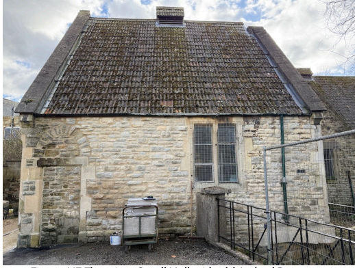
Fig 7 – NE Elevation: Small Hall with old Arched Doorway
