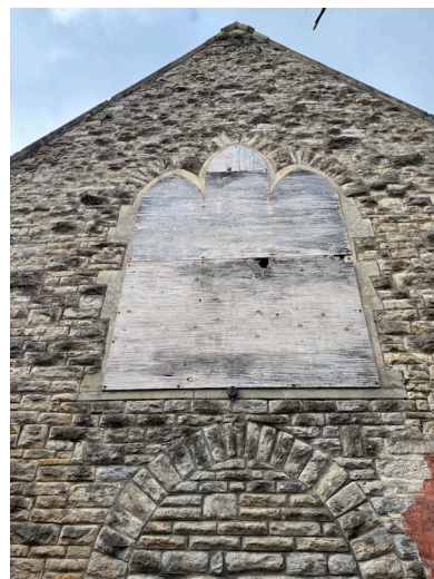
Fig 6 – SE Elevation Detail: Blocked Arch & Blocked Window
