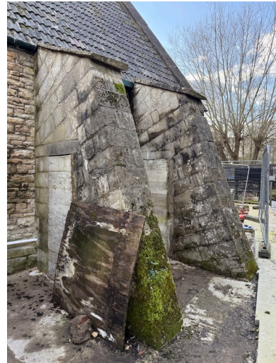
Fig 10 – NE Elevation: Existing Flying Buttresses
