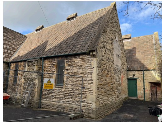
Fig 4 – SW to SE Elevation: Clay Pantile Roof & Condition
