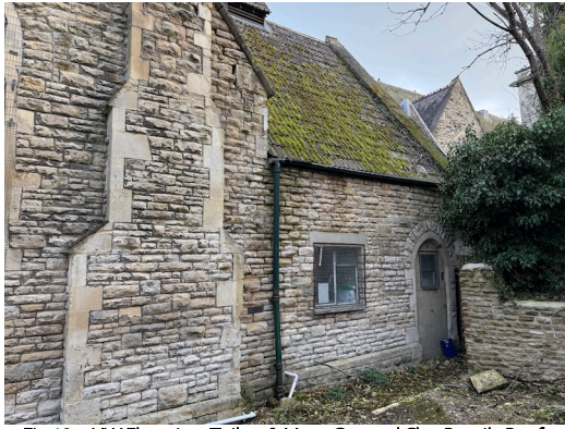
Fig 13 – NW Elevation: Toilets & Moss-Covered Clay Pantile Roof
