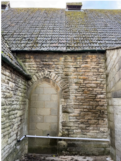
Fig 9 – NE Elevation: Small Hall Old Blocked Up Entrance
