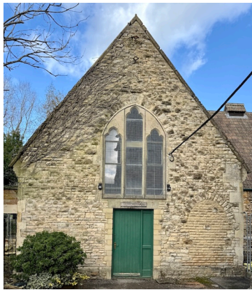
Fig 3 – SW Elevation: Main Entrance & Stone Mullioned Window
