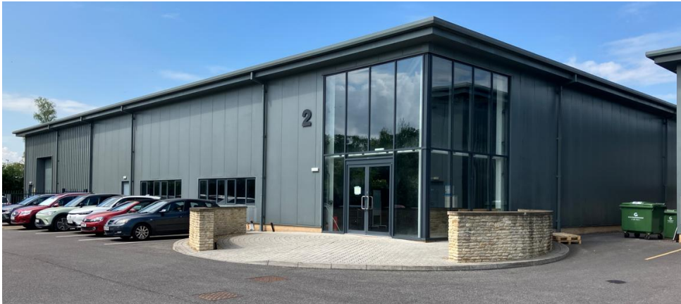
Figure 1 - photo of main South East elevation of Unit SP2
