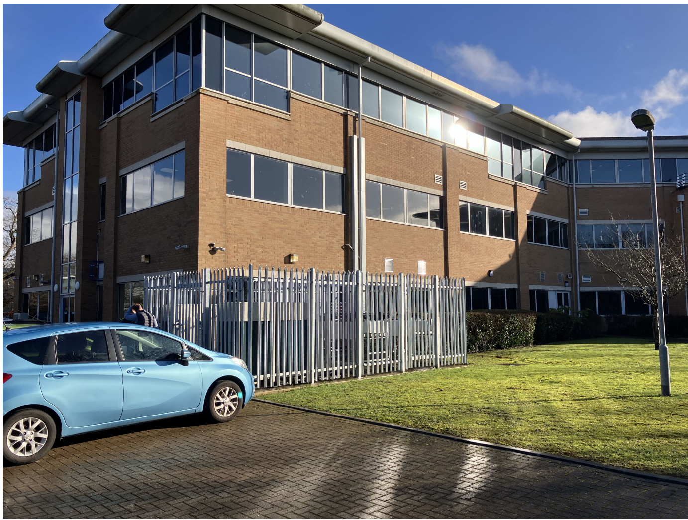
View of existing plant enclosure, with 2.4m galvanised steel palisade fencing surround
