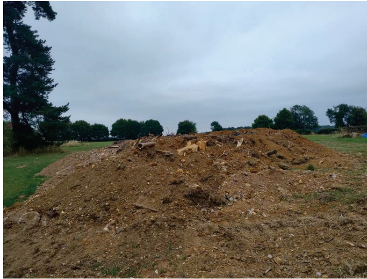
Figure 2: Spoil heap present due to current works
