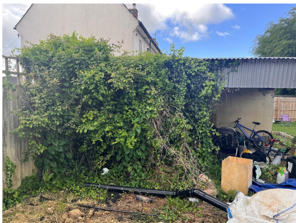
Photograph 3: Ivy and bramble growing on outside of lean-to
