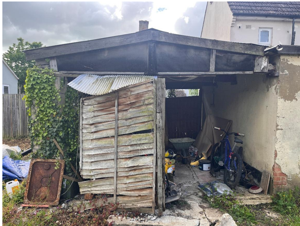
Photograph 4: North west elevation of lean-to
