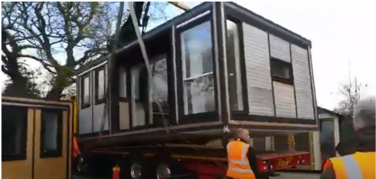
Figure 1 Removal of hybrid annexe by truck/hoist
