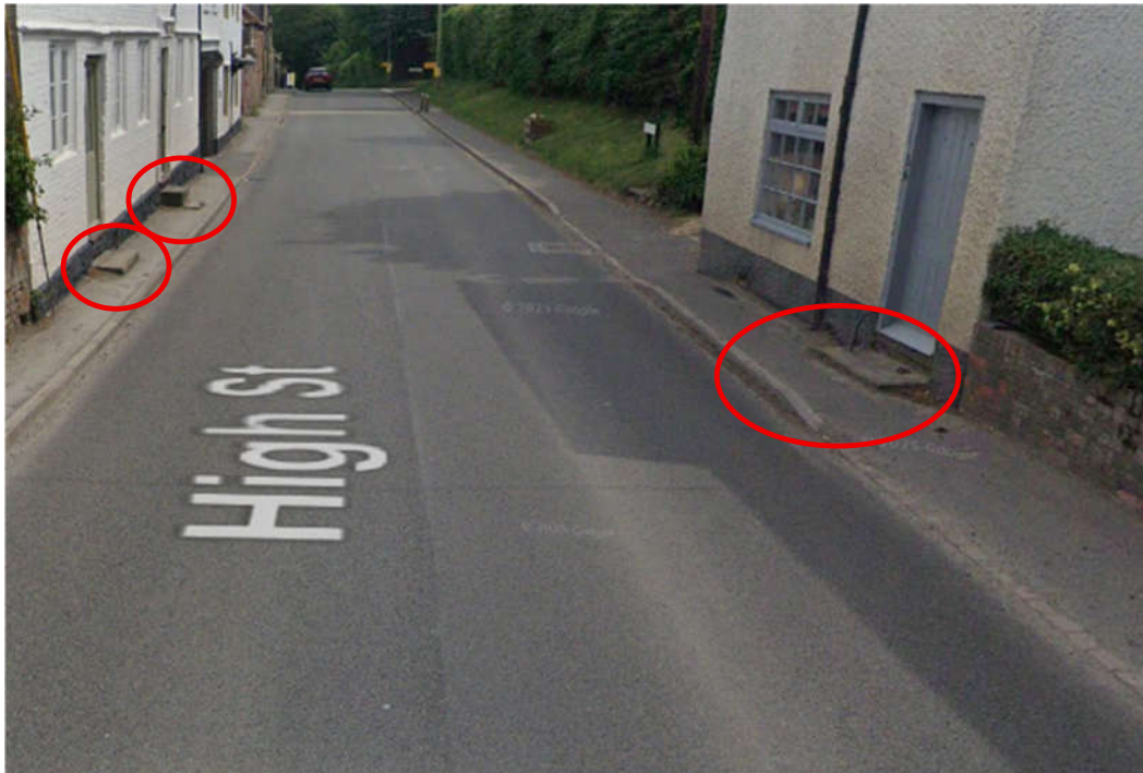
Figure 3.1 Footway interrupted by doorway thresholds (circled)
