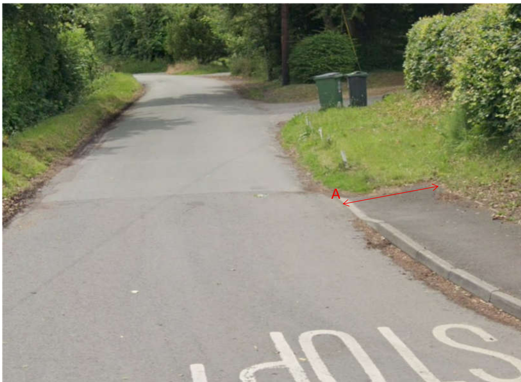
Figure 5.1 Footway Measurement on-site (1.5m)
