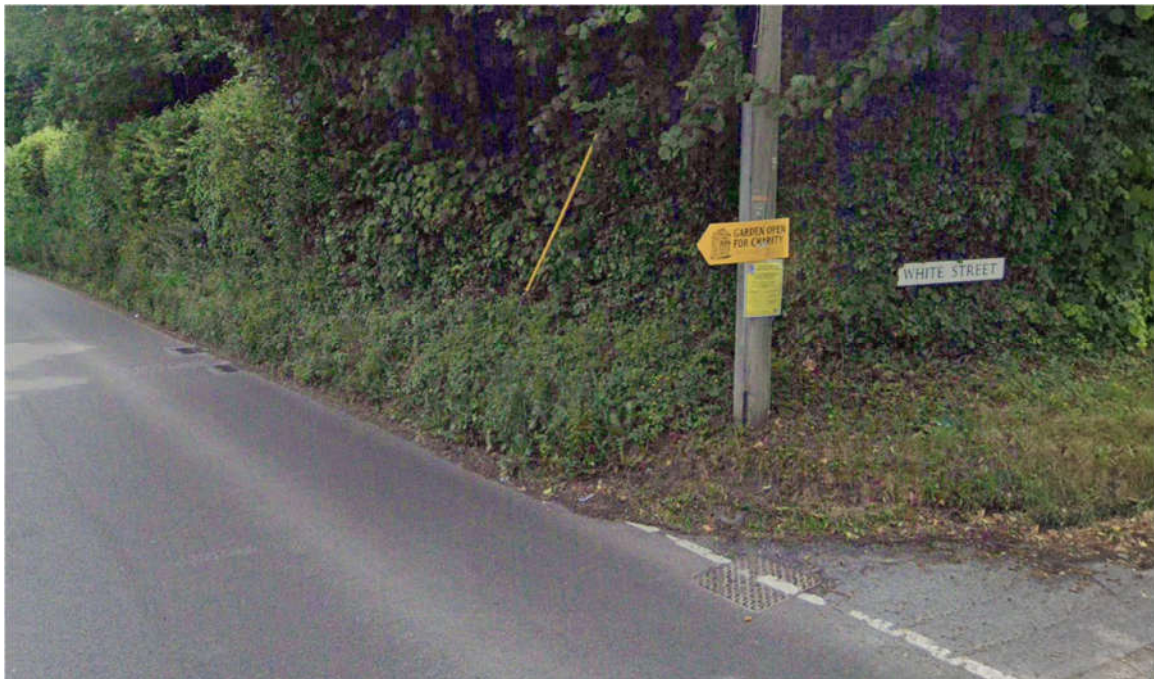
Figure 5.5. Highway verge is steep/near vertical and will likely preclude the visibility splay being achieved in the vertical plane
