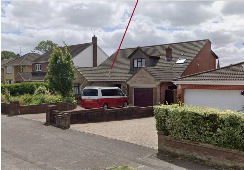
Front view of 20 Sadlers Mead, attic conversion (2 storey at rear) with dormer to front.
