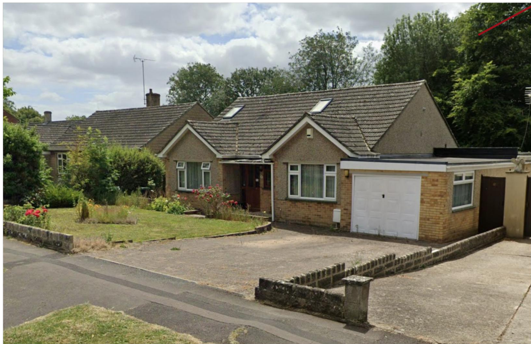
12 Sadlers Mead, attic conversion, as viewed from road frontage.
