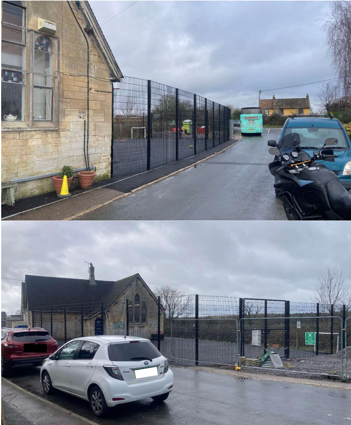
Figure 3: Images of the site from school lane and the unauthorised 3m high fence
