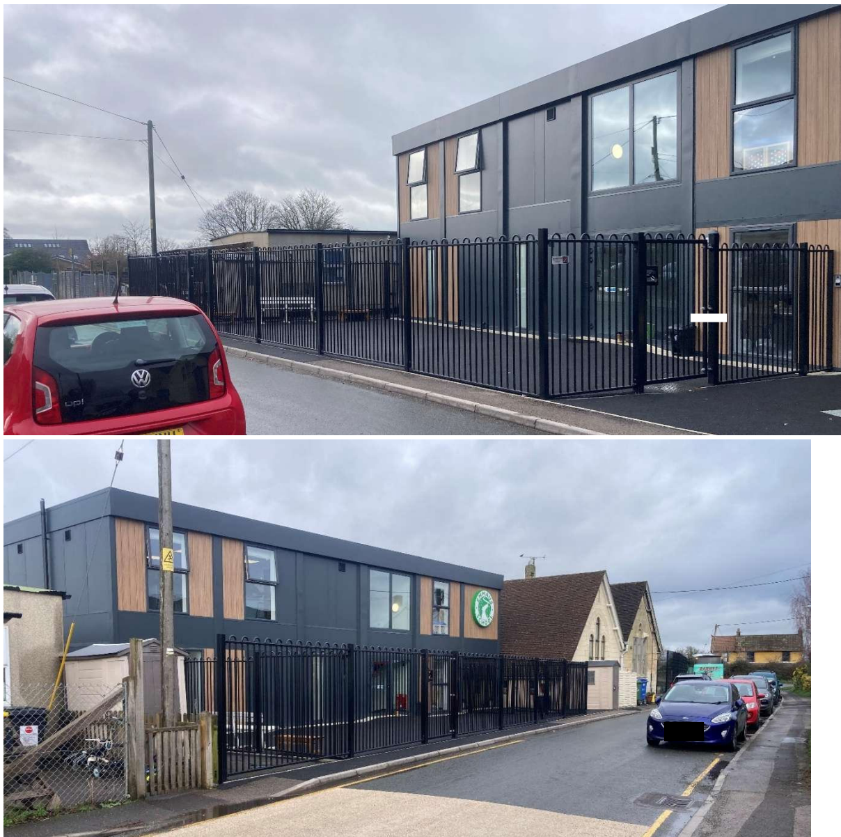
Figure 2. Views along school lane showing the 2m high metal rail fencing
