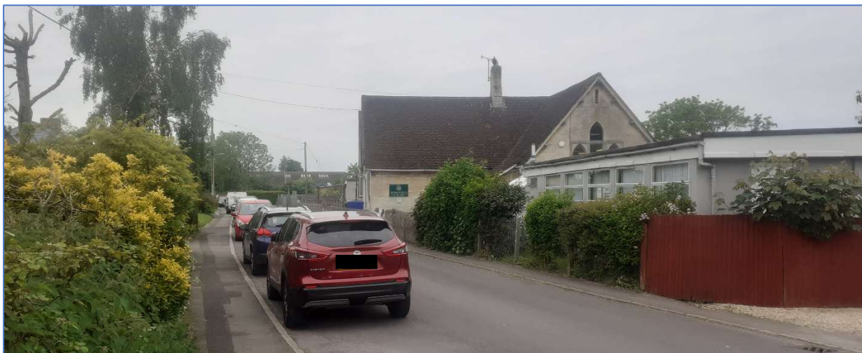
Figure 2: View of northern façade of building prior implementation of planning permission PL/2023/10641
