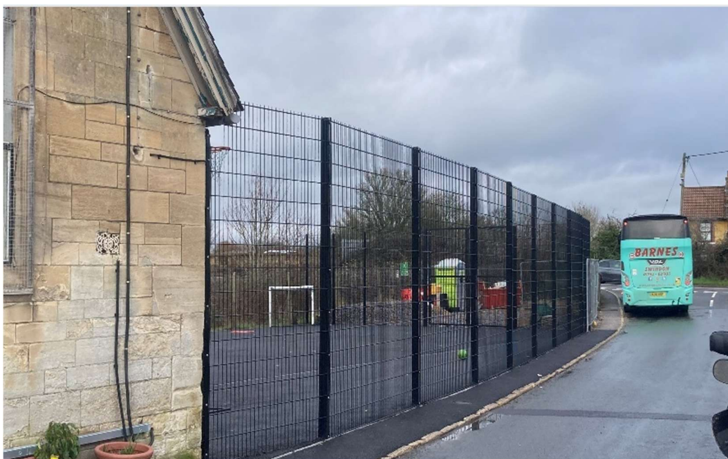
Figure 8: 3m fence enclosing playground – not supported by officers
