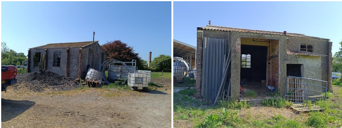
Photographs 1 and 2 – Former RAF building subject of application
