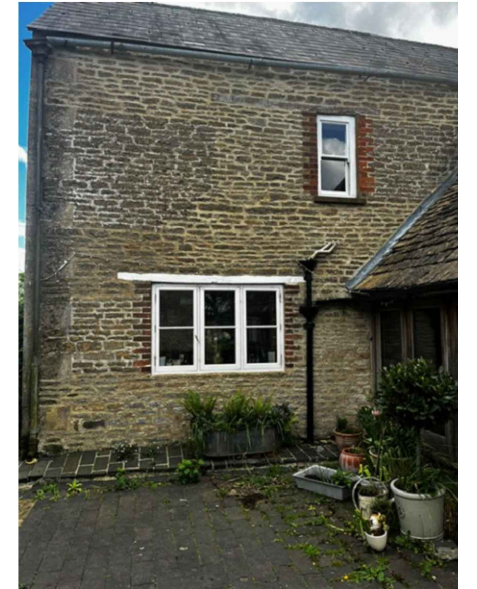
Existing down pipes and patio:
