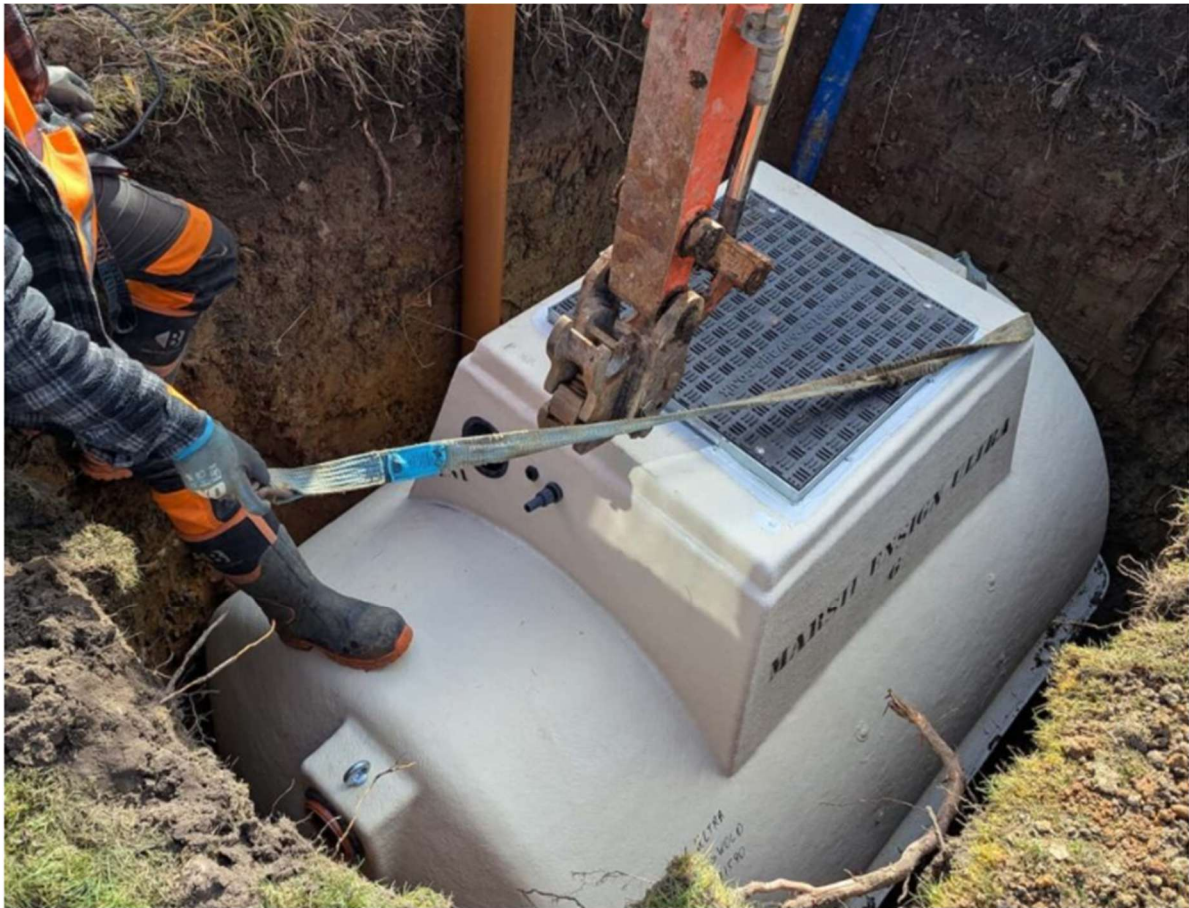
Figure 2: Example water treatment tank being installed
