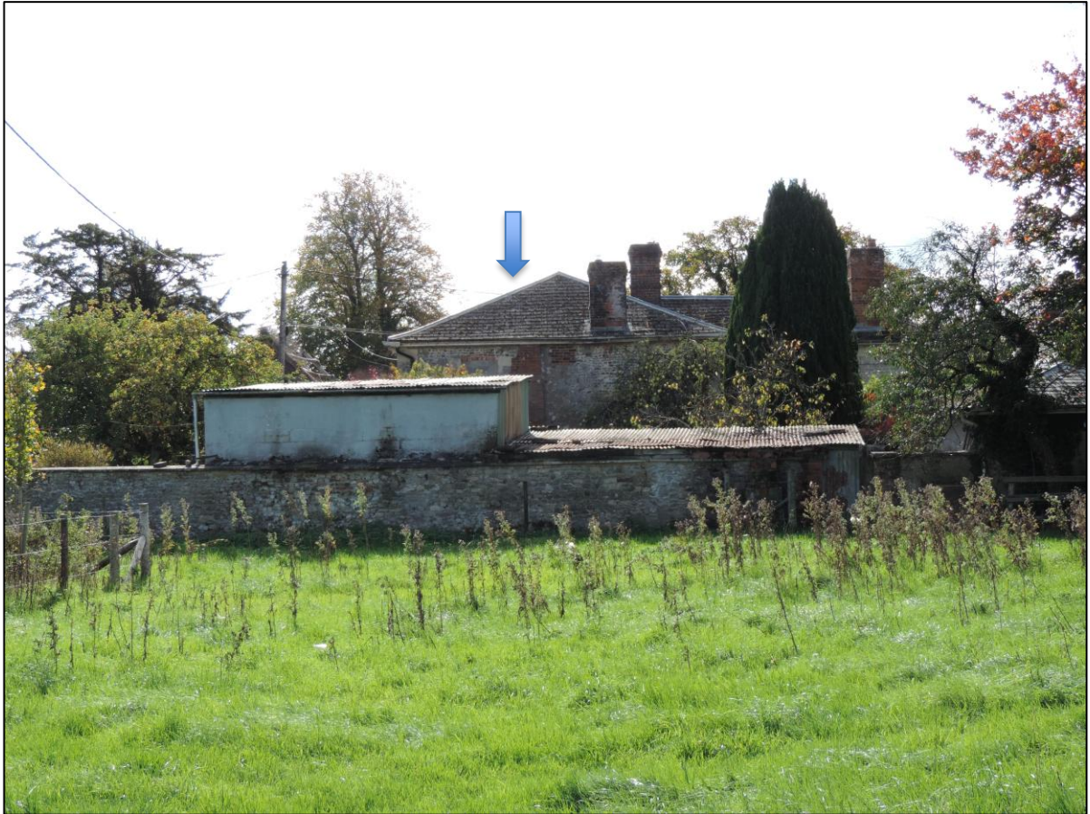
Photo 5 South facing view of the grade II listed Mill House from the Project Site. Property marked with a blue arrow.
