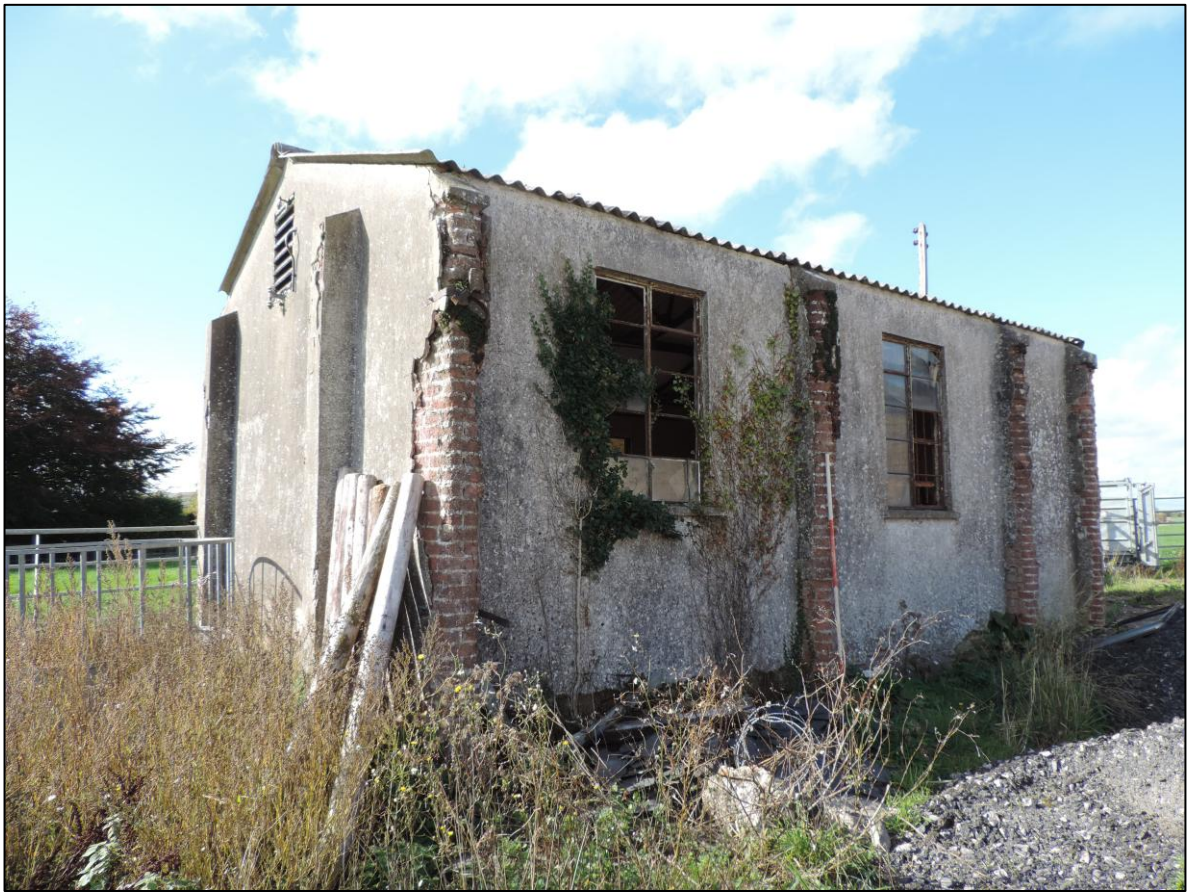
Photo 1 West facing view of RAF Alton Barnes temporary brick hut, erected 1941 (Scale 2m).
