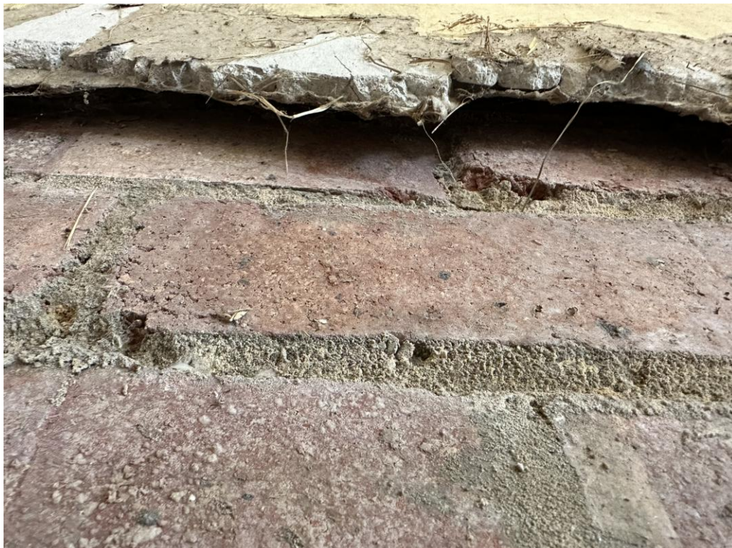
Photograph 4: Gap between plasterboard and brickwork.
