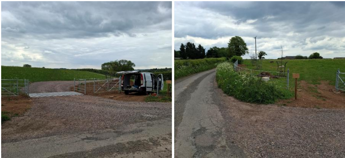
Figure 5: Works that have taken place so far when a site visit was made in May 2026.
