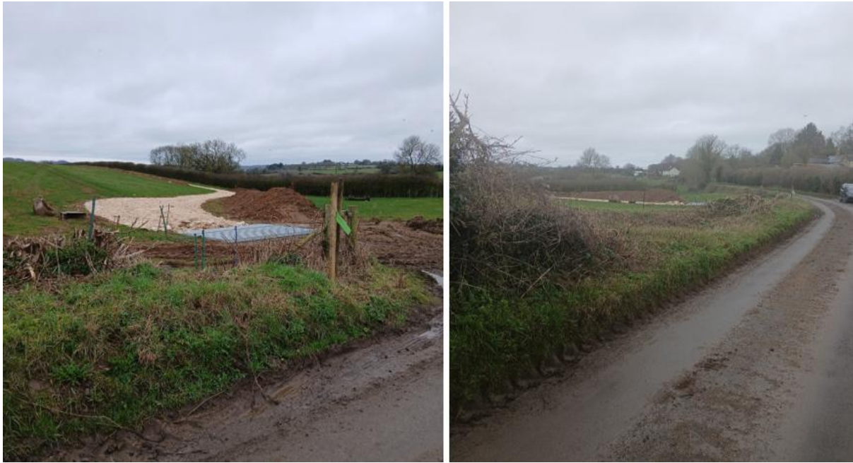
Figure 4: Works that have taken place so far when a site visit was made in February 2026.
