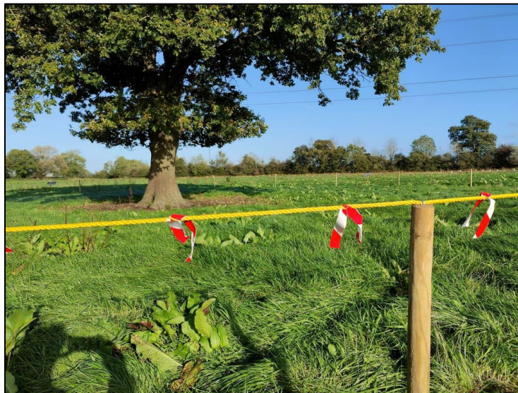
Figure 1: The tree protection fencing for this project could be as simple as coloured rope nailed to wooden fenceposts as shown in this image.
