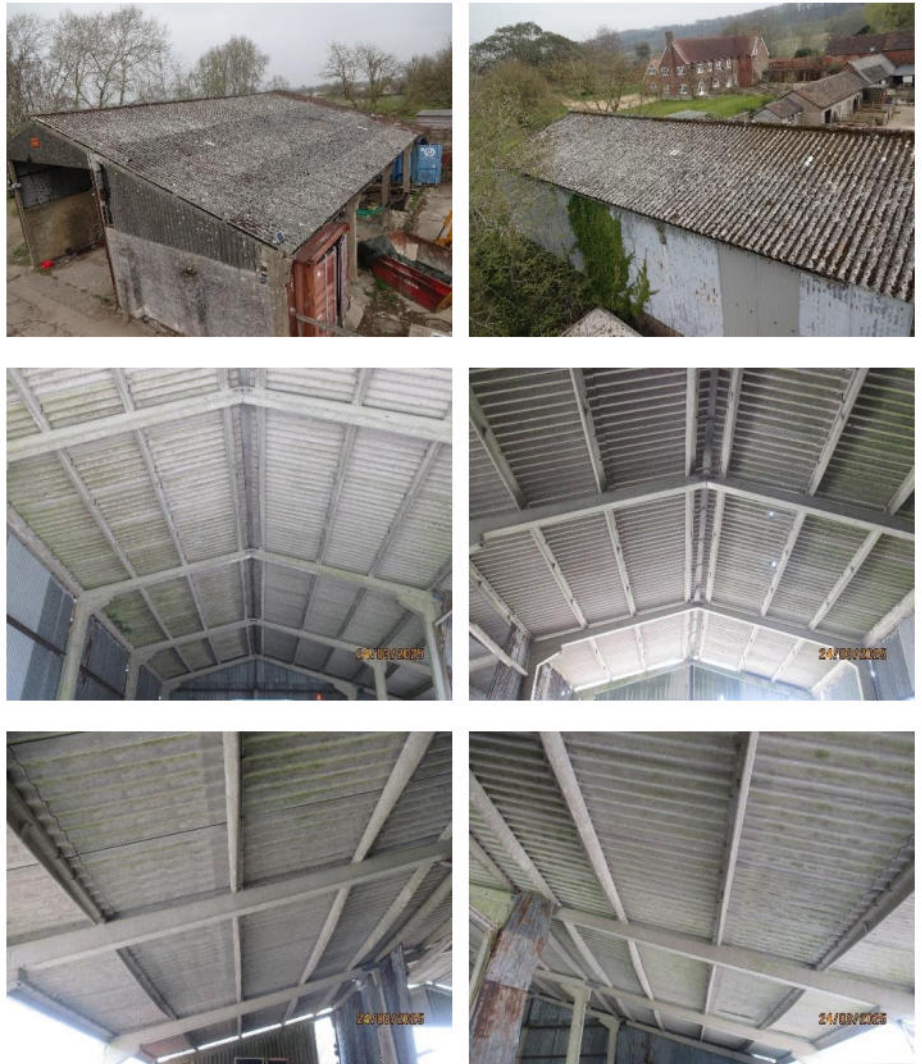
Images showing the barn and lean-to roof
