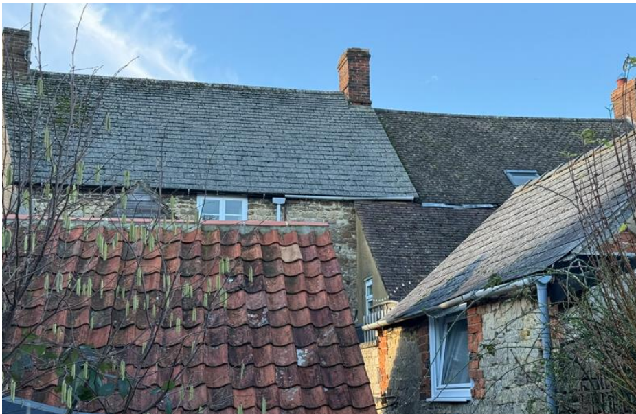
Photograph 9: Rear of No.49 & No.51 The Triangle
