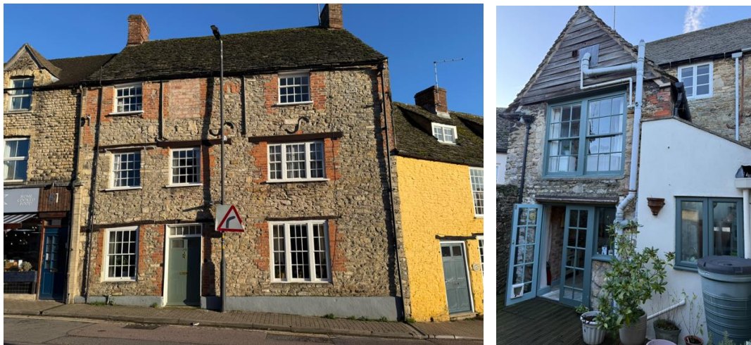
Photographs 1 & 2: No.49 The Triangle Front & Rear Elevations
