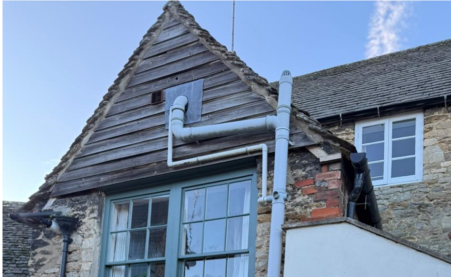
Photograph 7: Roof of Rear Two-Storey Extension
