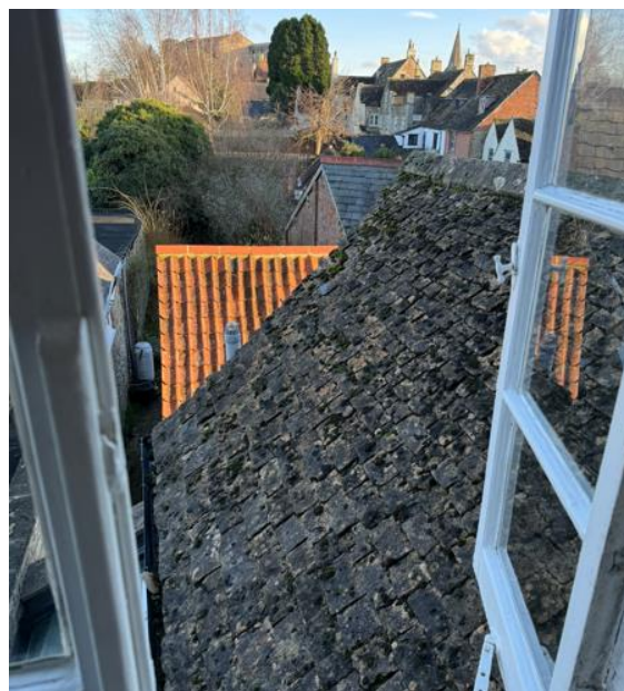
Photograph 6: Roof of Rear Two-Storey Extension
