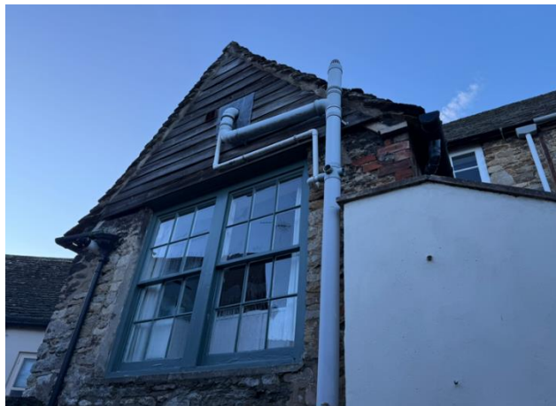
Photograph 5: Rear of No.49 The Triangle (close range)
