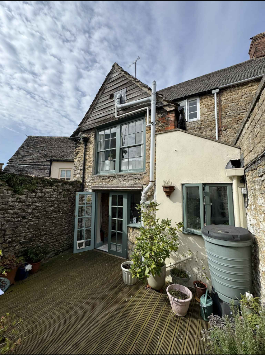
PHOTOGRAPH OF SOUTH EAST ELEVATION
