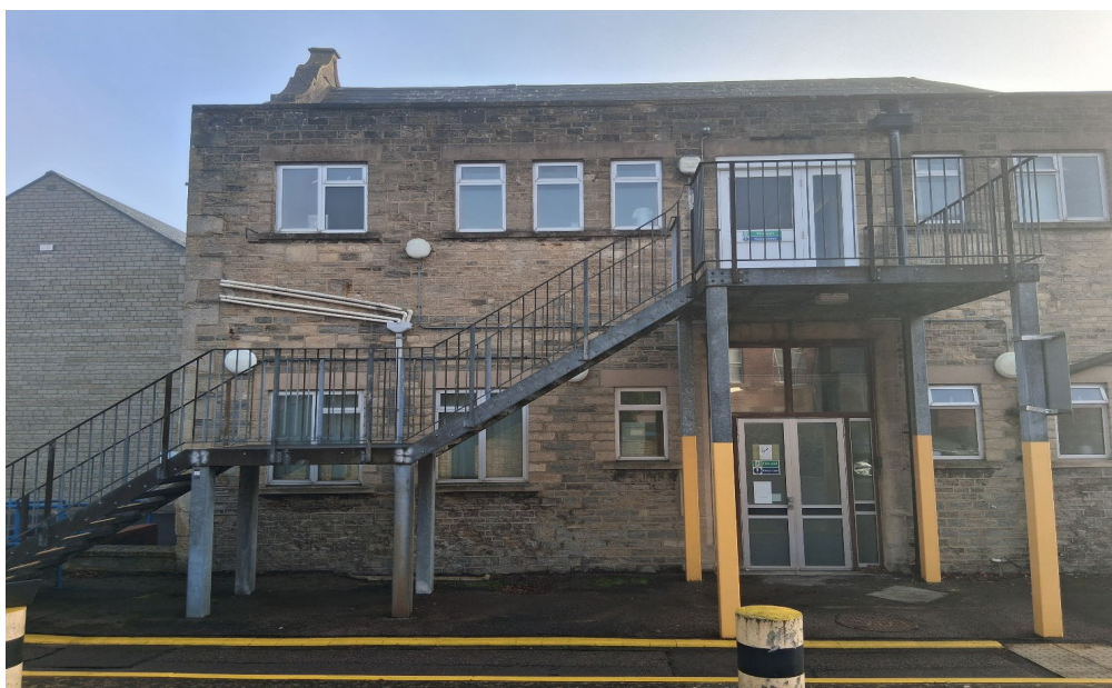
Fig 10: Typical existing condition, east elevation.
