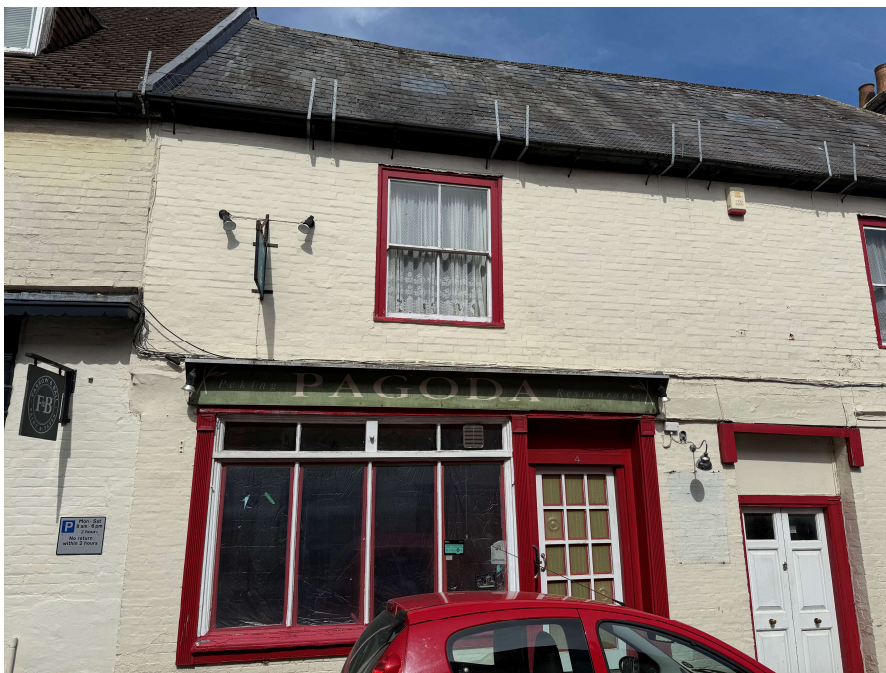
Existing Elevation and Signage
