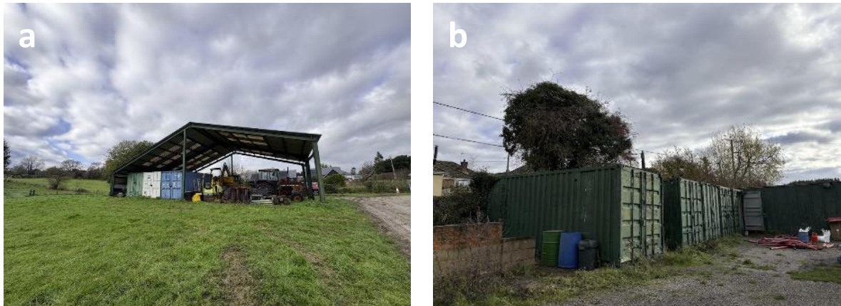
Figure 11. The building (a) and shipping containers (b) found on site (taken November 2025).
