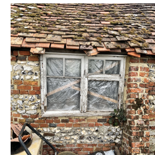
REPAIRS TO BRICKWORK & FLINT
