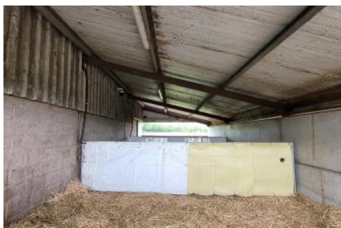
Photo 9: B2 – An internal view of the lean to element.
