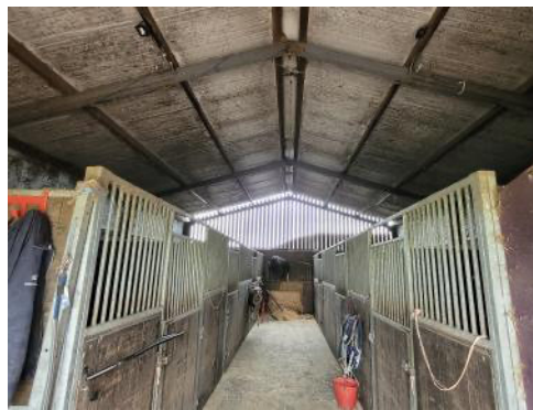
Photo 8: B2 – An internal view of the main structure.
