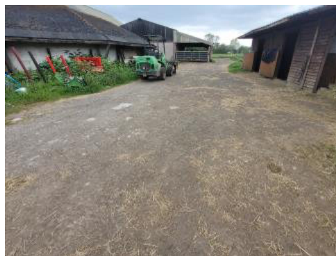
Photo 16: Compacted gravelled surface surrounding the buildings.
