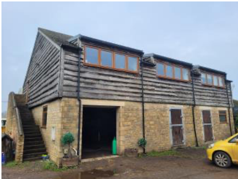
Photo 3: The east facing front elevation of B1.
