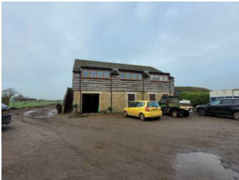
Photo 1: A view of the surveyed building B1 from the east of the yard.
