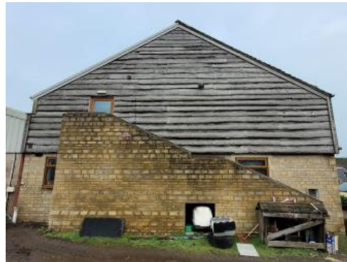
Photo 4: B1 - The southern gable end with external steps to the first floor.
