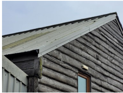
Photo 2: B1 - metal sheet clad roof pitch.
