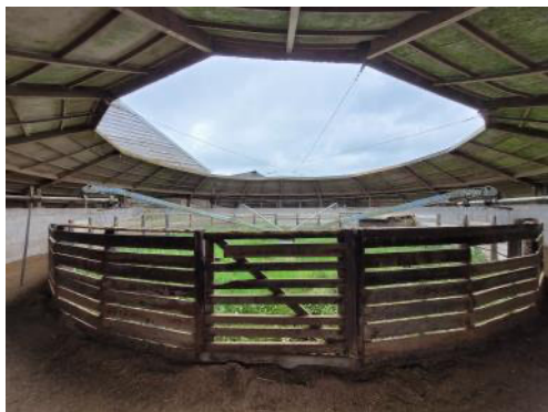
Photo 13: B4 – An internal view of the structure.
