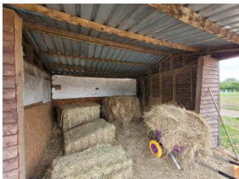
Photo 11: B3 – An internal view of the structure.
