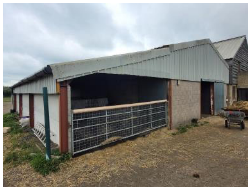
Photo 7: A view of the surveyed building B2 from the south-west of the yard.
