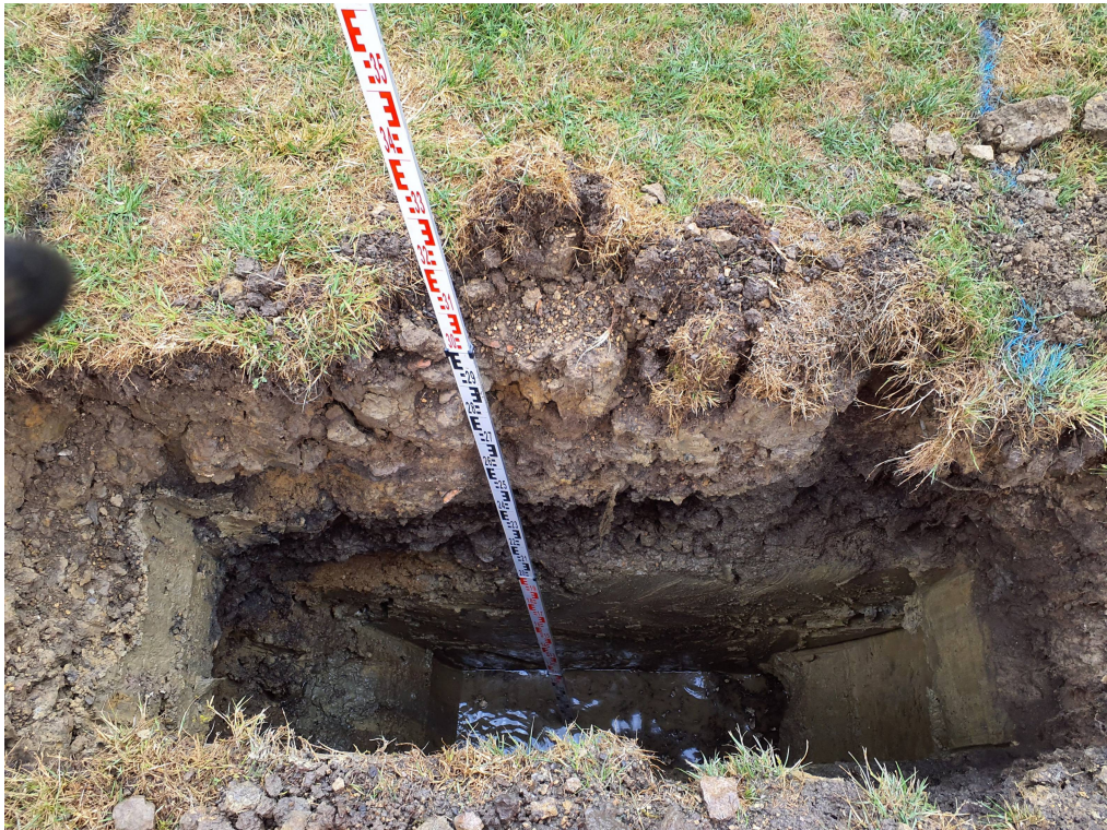
View looking west (before pit extended south to join TP05A).
