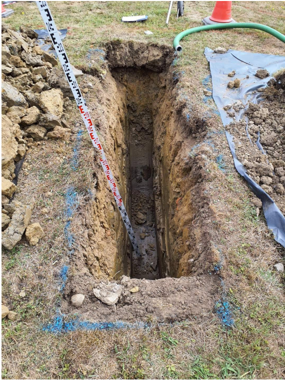
Excavation prior to commencing soakaway test.
