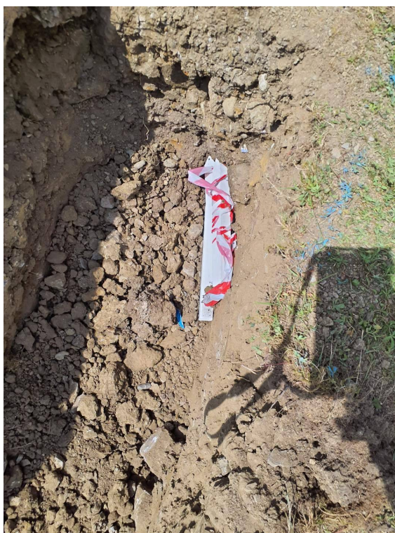
Pipe protected when backfilled using wooden pegs.
