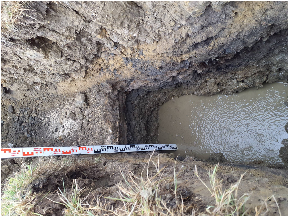
View south showing edge of concrete slab.
