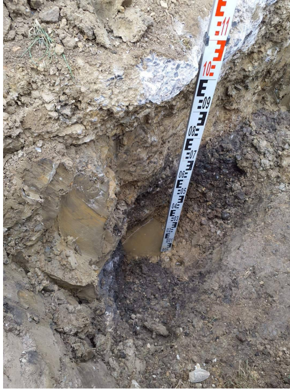
Concrete foundation tapering in towards building.
