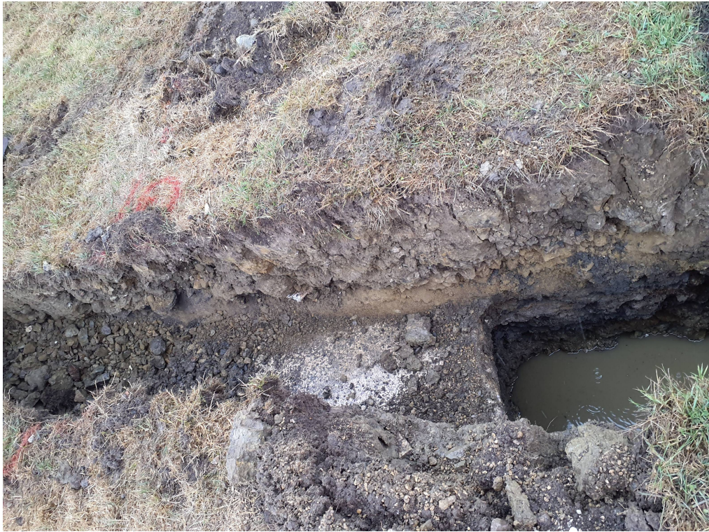
Edge of concrete exposed at northern end of pit (which bounds TP05B).
