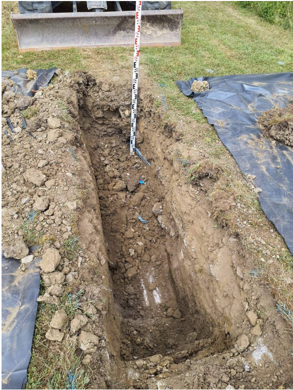
Excavation. Concrete in base, pipe in NW corner.
