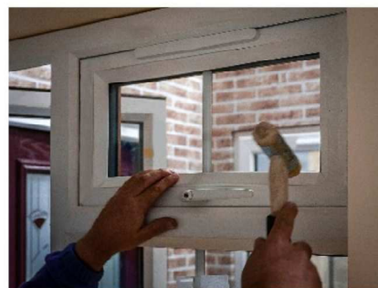
Example of beads being carefully tapped into place
