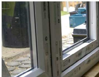
Bridge packers in position
