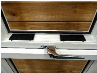
Bridge packers in position
