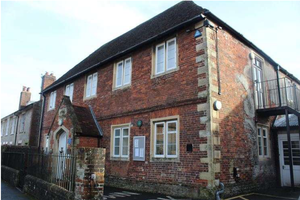
Fig 1 – Front elevation of building to North Row
