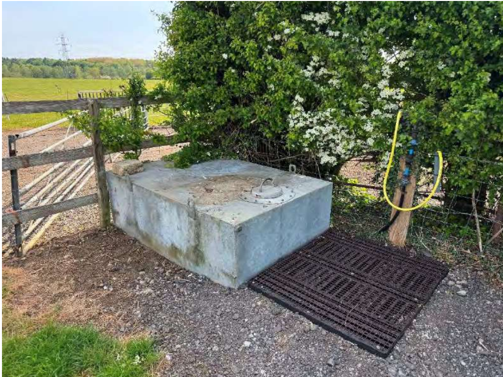
Photo 12: Presumed water supply and waste disposal point in east corner of Field 1.
