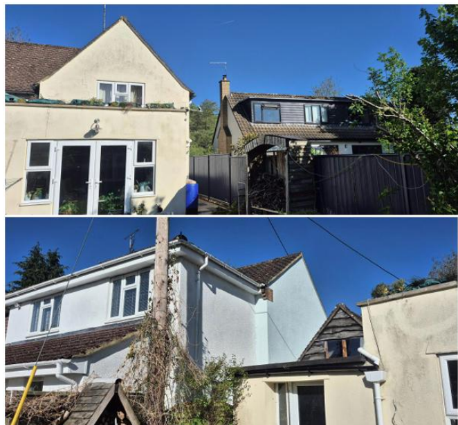
Figure 11: site photos (top) site & no.4 (bottom) site & no. 2
