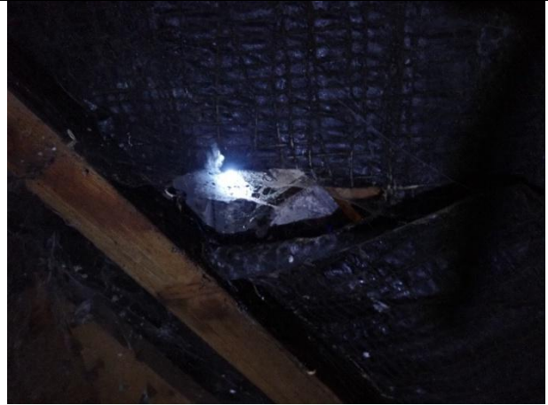
Photograph 14: Internal void, gaps in bitumen felt.
