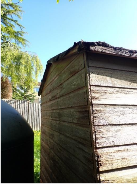
Photograph 18: West elevation of the shed.
