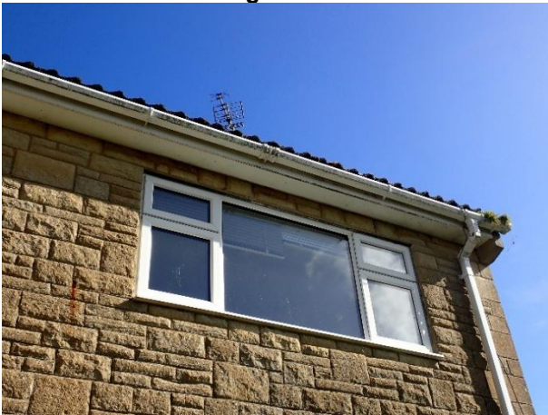
Photograph 9: Soffits on southern elevation of the roof.
