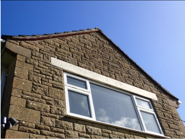
Photograph 7: Dormer extension, south facing gable.
