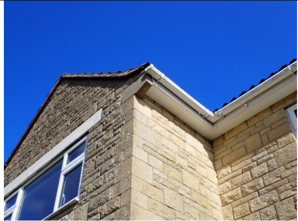
Photograph 8: Dormer extension, south facing gable.
