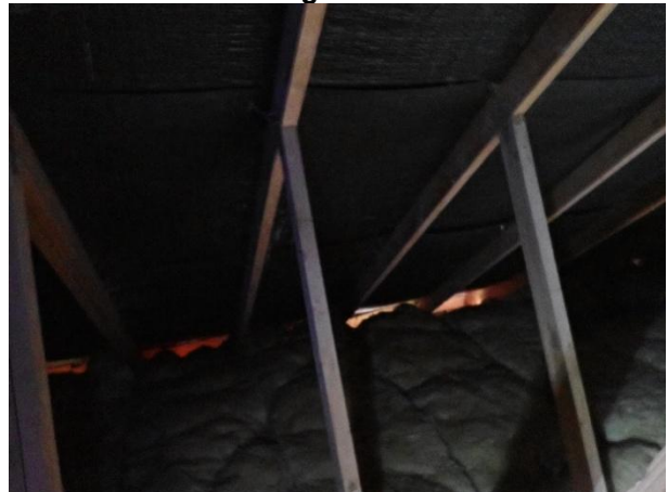
Photograph 12: Internal loft void showing light ingress.
