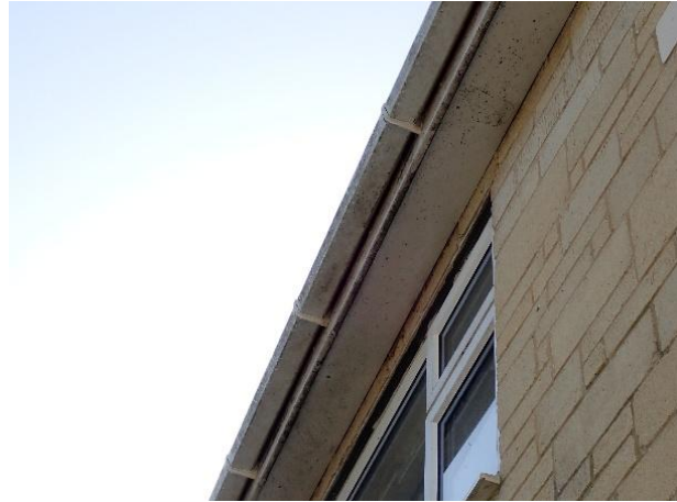
Photograph 4: Soffits on northern elevation.
