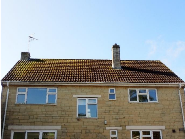
Photograph 1: The northern elevation, showing both chimneys.
