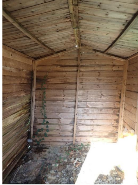
Photograph 19: Shed internal space.
