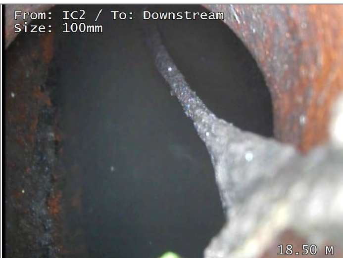
End of survey: Entered the Main sewer.
