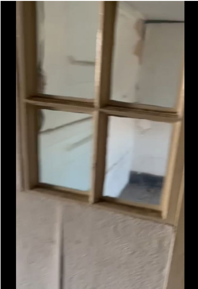
Photo 8 - Non-historic sidelight next to doorway
