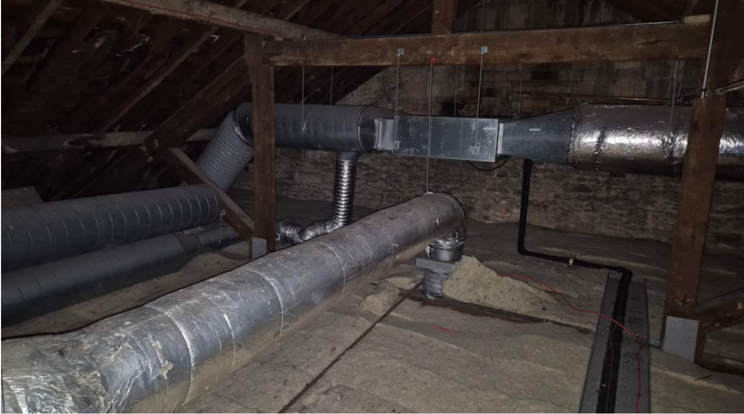
Image of current arrangement in roof void
