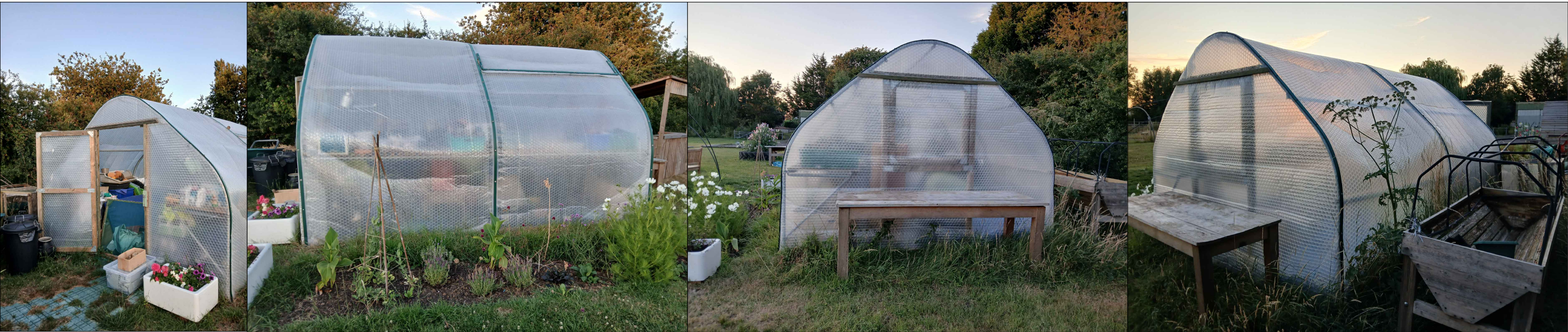
PHOTOGRAPH 5 NORTH ELEVATION PHOTOGRAPH 6 WEST ELEVATION PHOTOGRAPH 7 SOUTH ELEVATION PHOTOGRAPH 8 EAST ELEVATION
