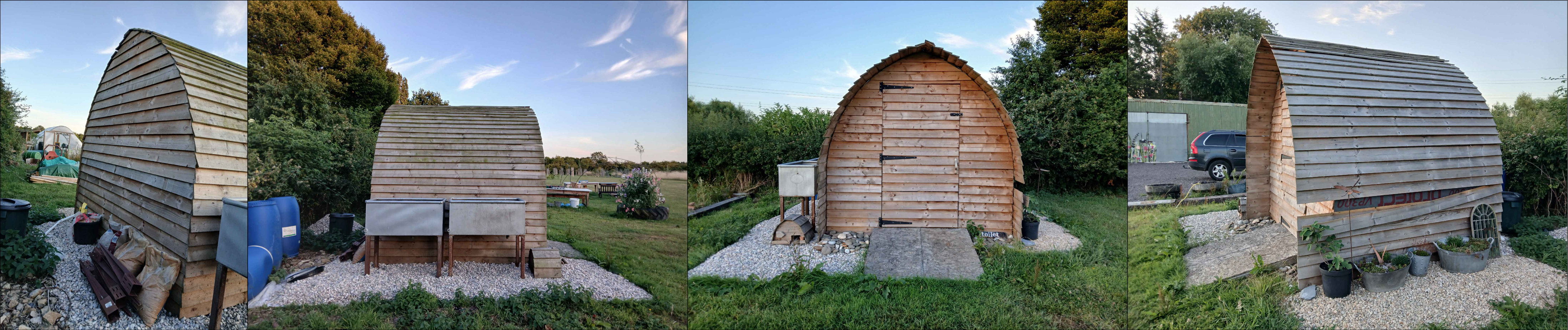
PHOTOGRAPH 1 EAST ELEVATION PHOTOGRAPH 2 NORTH ELEVATION PHOTOGRAPH 3 WEST ELEVATION PHOTOGRAPH 4 SOUTH ELEVATION
